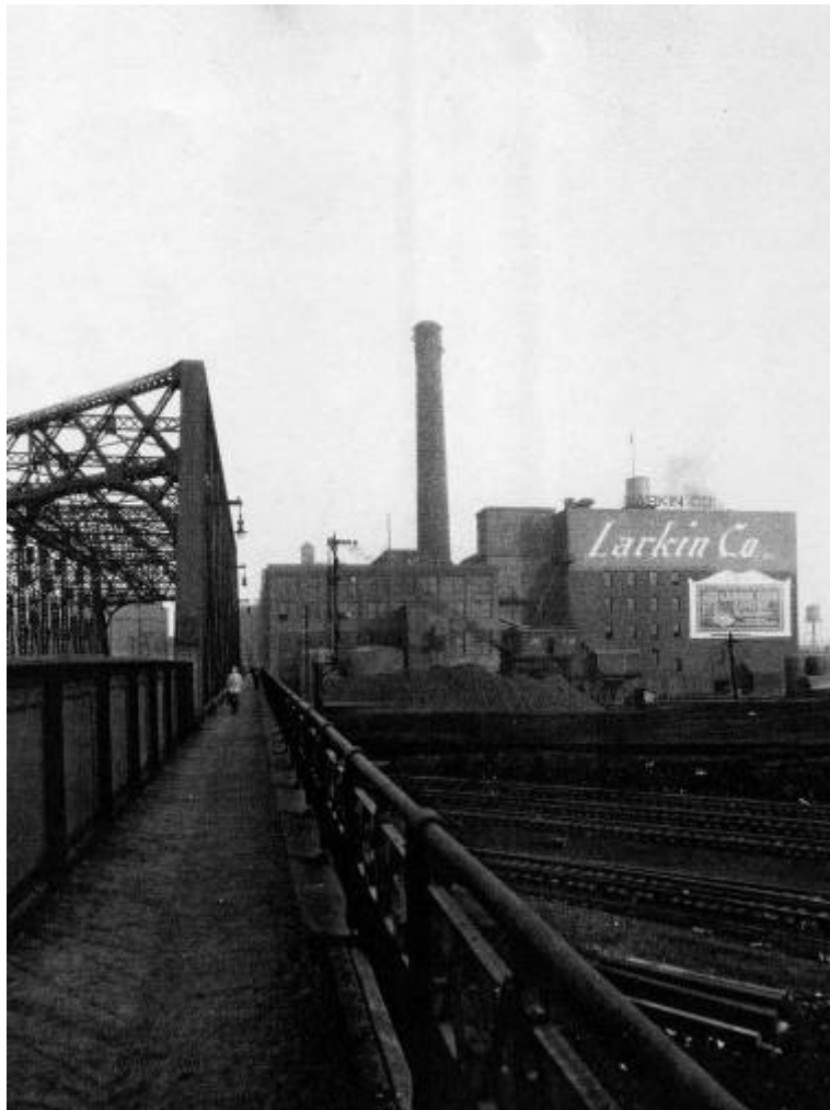
Figure B-19: Seneca Street viaduct, looking east towards the Larkin Company, undated
