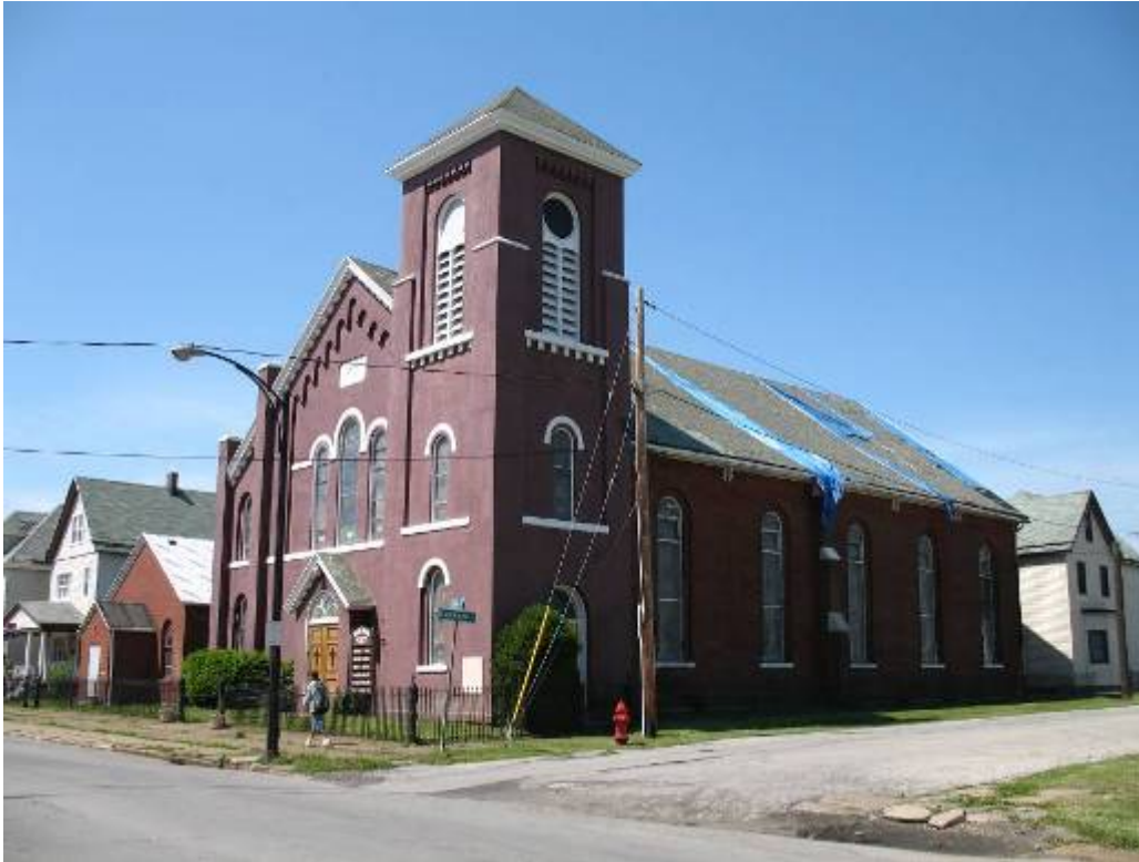
Figure C-11: 688 Swan Street ((former St. Matthew's German Evangelical Church) An excellent example of church architecture
