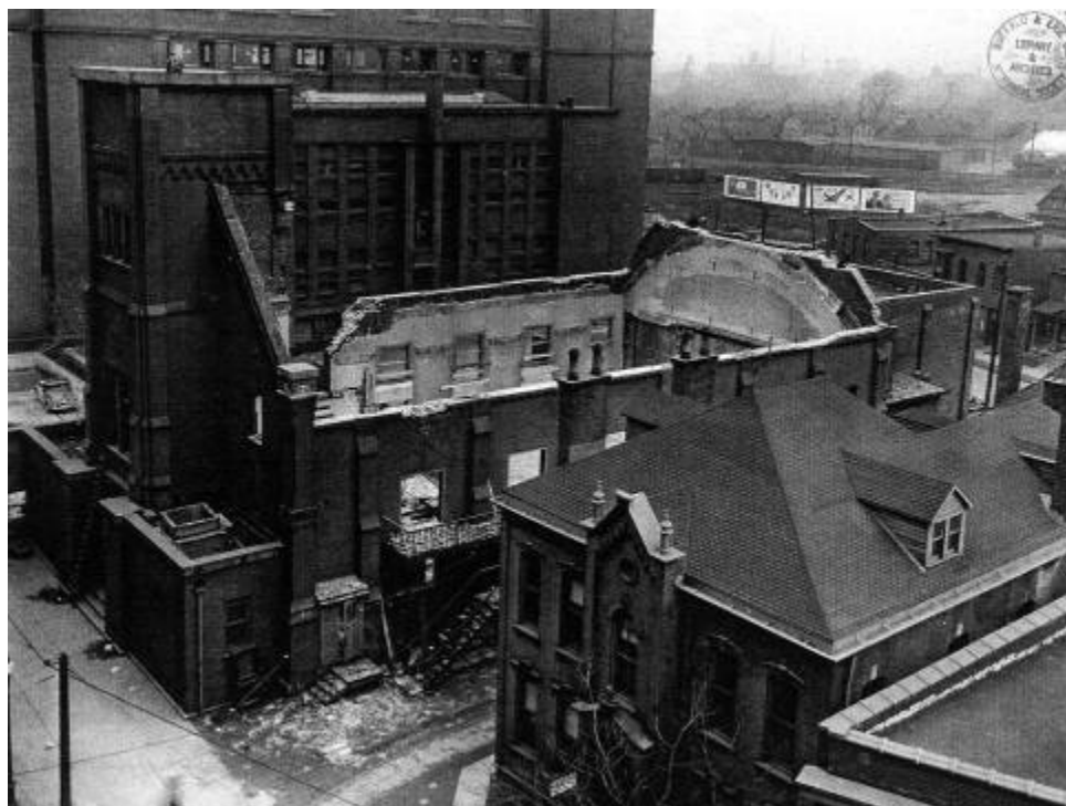
Figure B-6: Demolition of the Larkin Auditorium/ former Sacred Heart Church, ca. 1937
