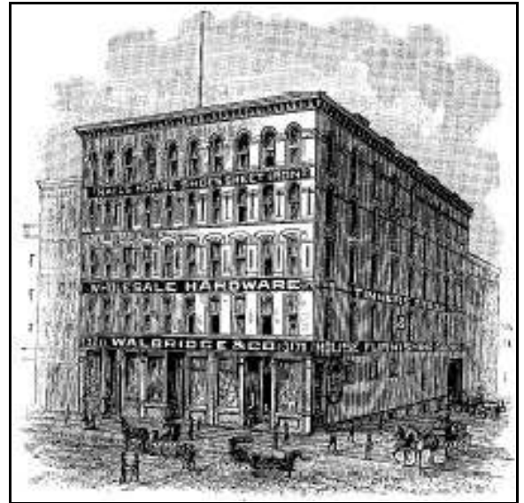
Walbridge & Co. Hardware on Washington St.
