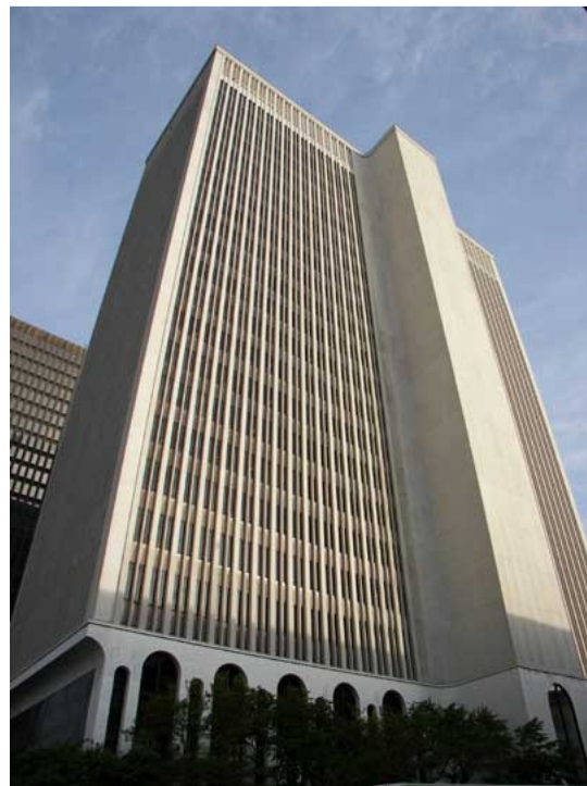
Figure 9. One M&T Plaza's Washington Street central service core serves as the building's spine.
