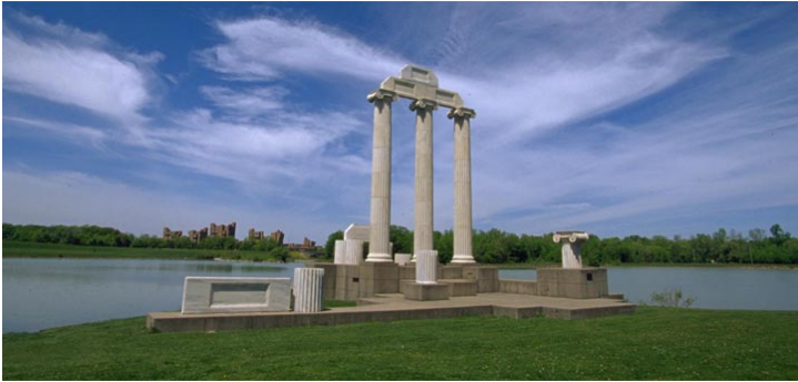
Figure 21. The columns from M&T's former headquarters are installed at Baird Point on the University at Buffalo's north campus.
