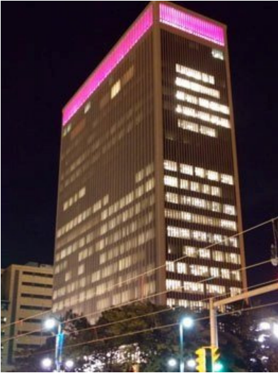
Figure 20. For special events, M&T Plaza's uppermost floor, separated by a horizontal white-colored band, is dramatically lit at night with appropriate colors.
