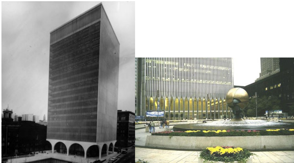
Figure 7. One M&T Plaza owes structural and appearance similarities to Yamasaki's 1962 IBM Building in Seattle (left) and 1963 World Trade Center in New York City (right).
