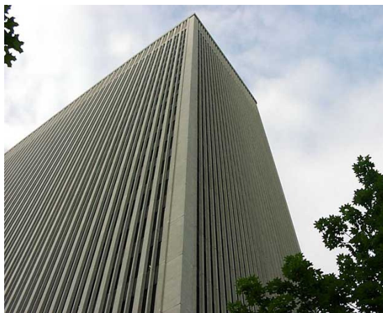
Figure 12. One M&T Plaza's white exterior contrasted with other Buffalo buildings covered in soot during the 1960s. The M&T building's visual upward thrust is accomplished through its use of continuous exterior structural columns and 4,000 narrow floor-to-ceiling windows.
