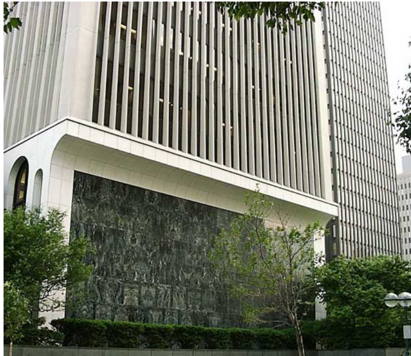
Figure 14. One M&T Plaza rests on a 35-foot first story base, covered with white and green marble panels and tall arched windows.
