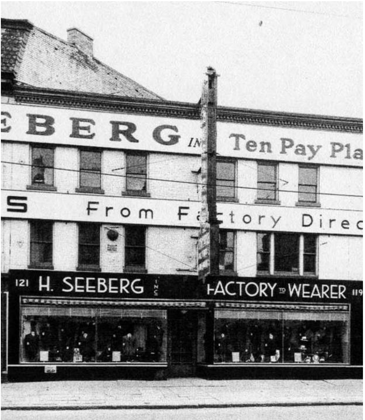
Detail, the H. Seeberg Building (121 and 119 spaces), ca. early 1940s Note the modest dentilated continuous cornice and the sleek storefronts.
