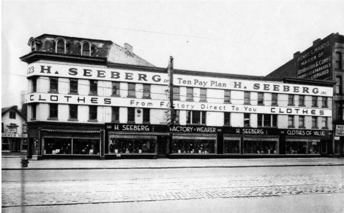
The H. Seeberg Building, seen from Genesee Street ca. 1940
