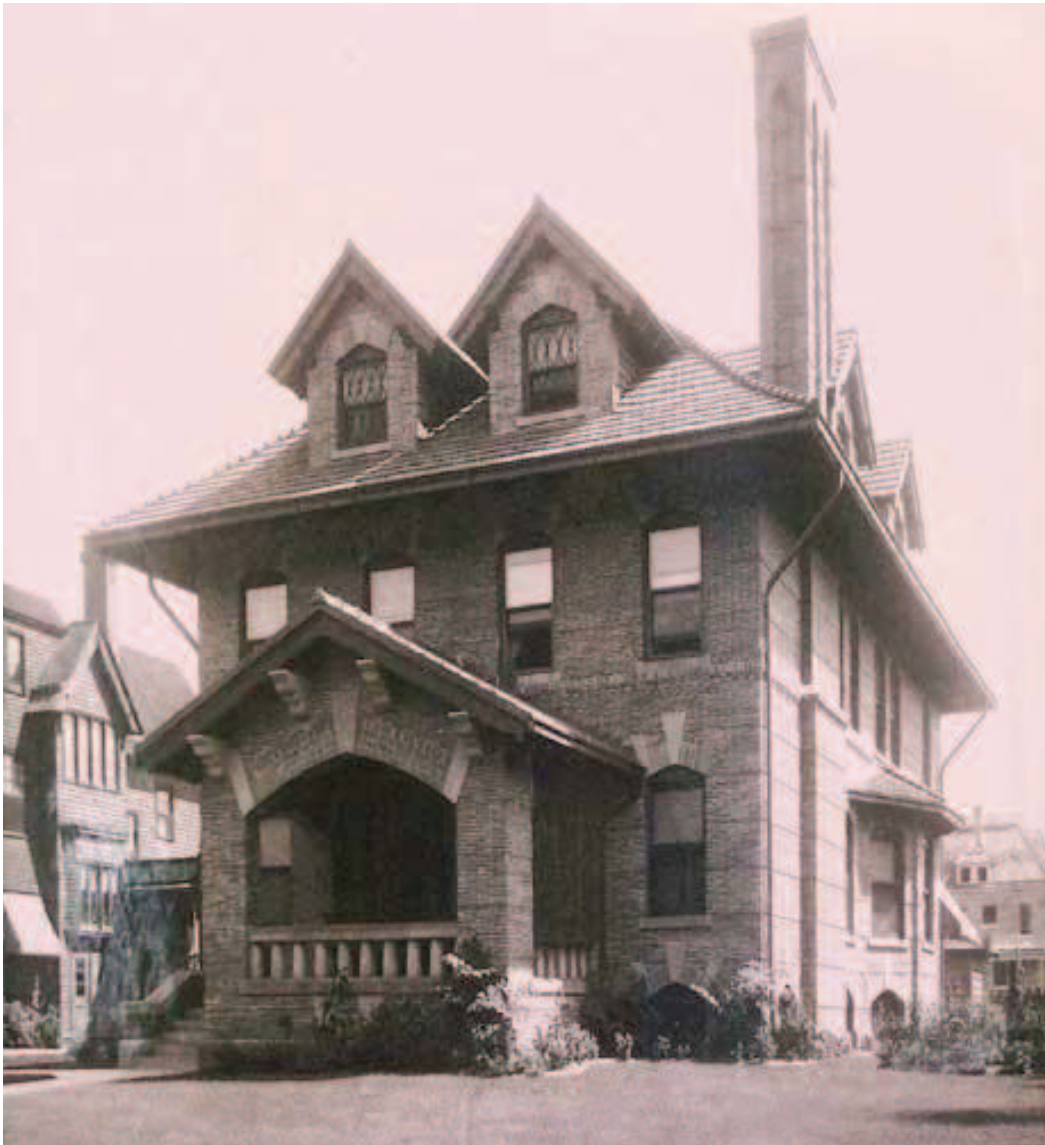
Edward H. Webster House, 781 West Ferry, ca. 1908
