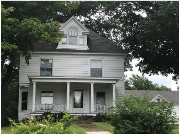
Figure 2-39: (left) 8 Prospect Street built ca. 1900 Source: CBCA
