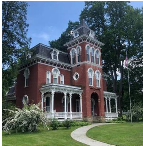
Figure 2-36: 21 Pearl Street built 1871 Source: CBCA
