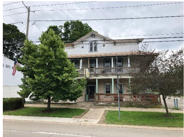
Figure 2-20: Main Hotel at 14 Main Source: CBCA
