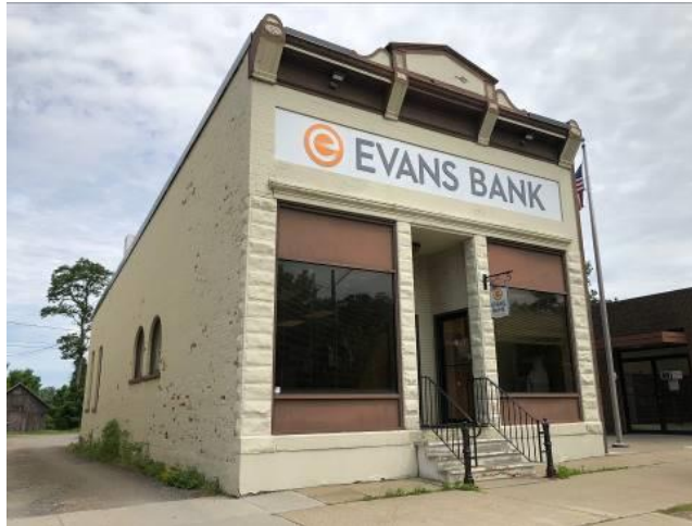
Figure 2-18: 25 Main Street built 1881 Source: CBCA
