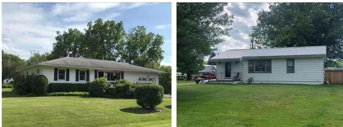
Figure 2-43: (left) 7 Swan Street built in ca. 1960 Source: CBCA
