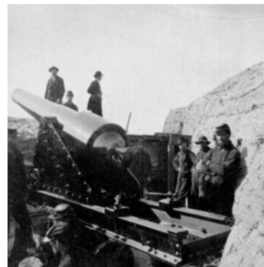
A 200-pound Parrott rifle in Fort Gregg on Morris Island, South Carolina, 1865
