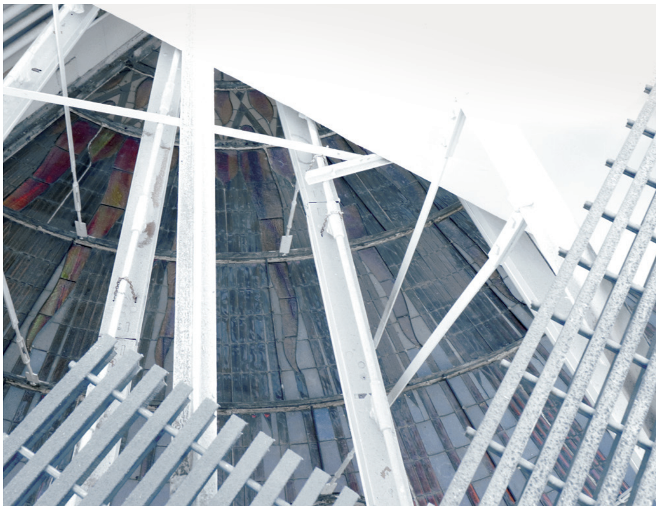
Figure 14: The Sunburst strut support for the steel bands; Photo: Bedson, 2019
