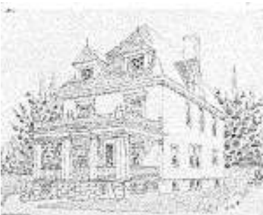
House built by Fred. W. Hudson, similar to 288 Hudson Street. Buffalo and Its Points of Interest, 1896.
