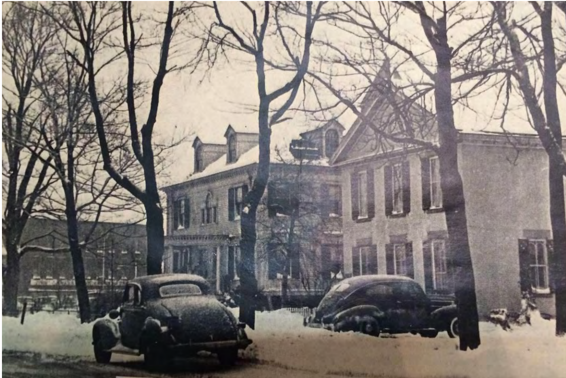
Potter-Eaton House at its original location on Broadway Street (photo courtesy of Lancaster Historical Society)
