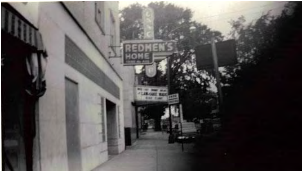
46-50 Central Avenue, ca. 1956 (photo courtesy of Lancaster Historical Society)
