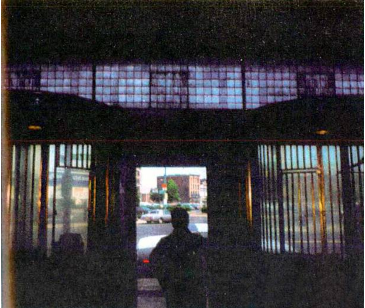
(13) Interior of 87 Genesee retail space, looking north, 1980 (John Conlin, photographer) Notice how light-filled the commercial spaces were following the 1914 alterations done by Colson-Hudson. This image highlights the ample storefront display windows as well as the Luxfer prism transom above.
