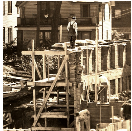
Music Hall under construction, 1939.
