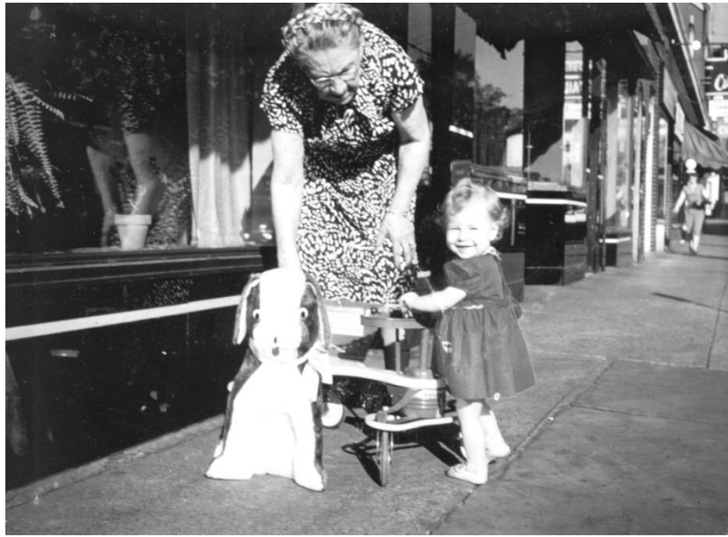
Figure 12. The black Vitrolite glass with white band can be seen on ground level. Photo from 1951. Ardie Bausenbach.
