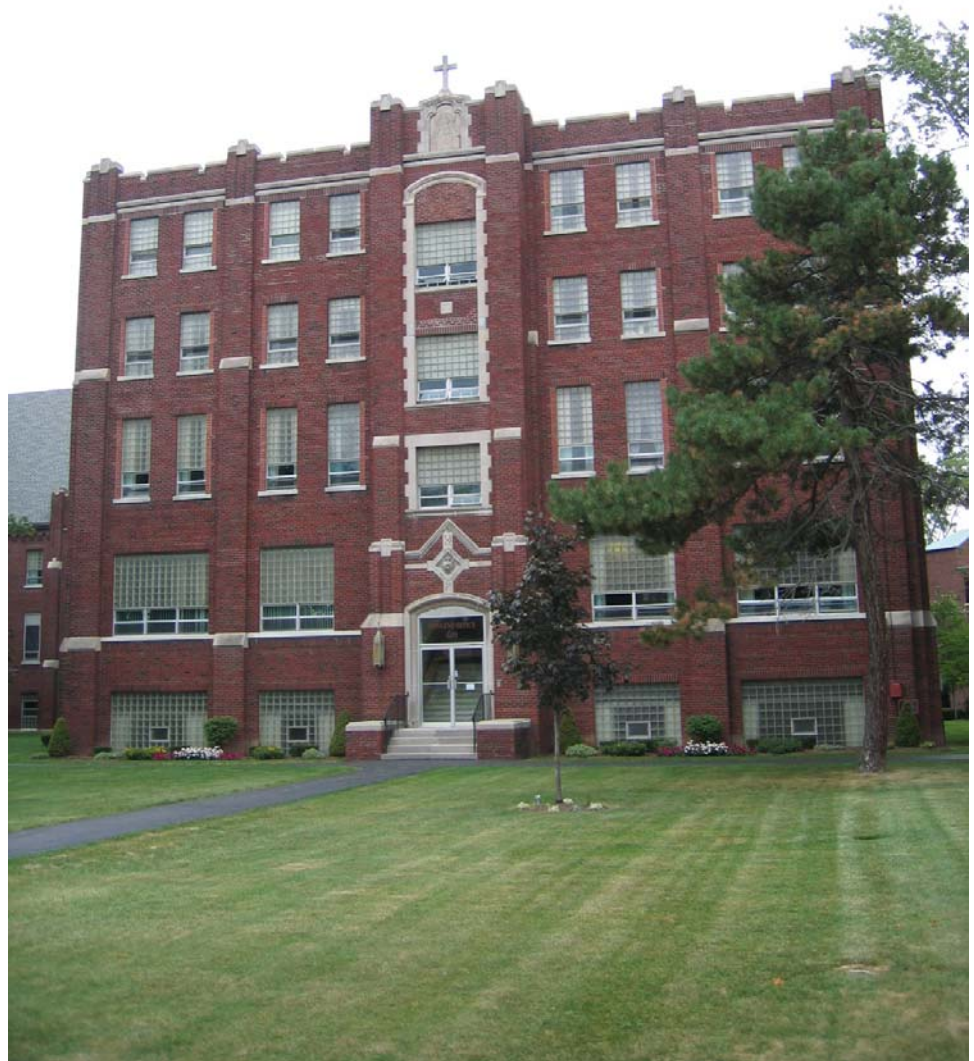
note non-original glass block windows which were removed
