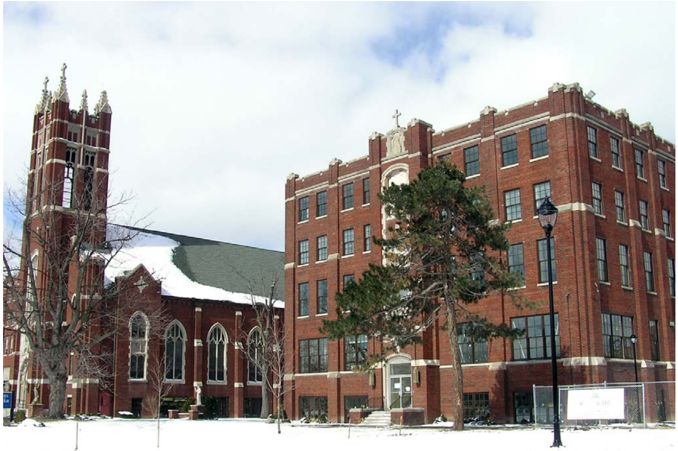
note window replacement complete – new units designed to match original configuration
