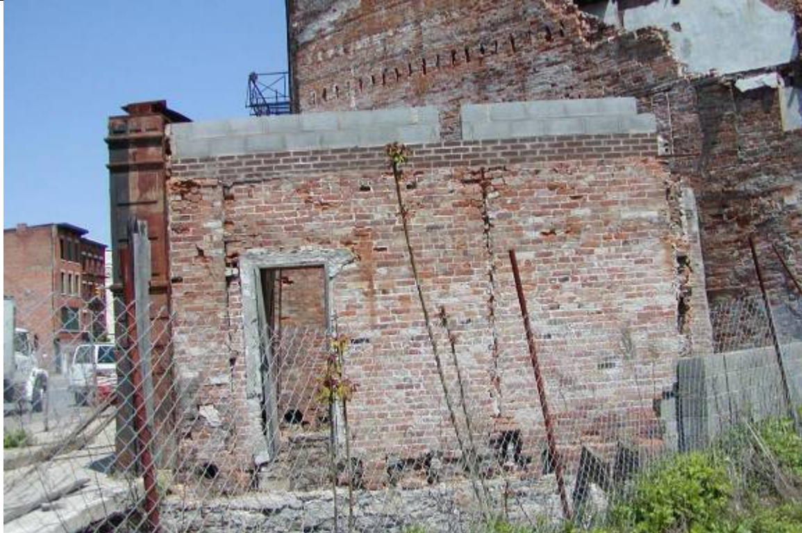
(12) 85-87-89 Genesee Street (west elevation)
