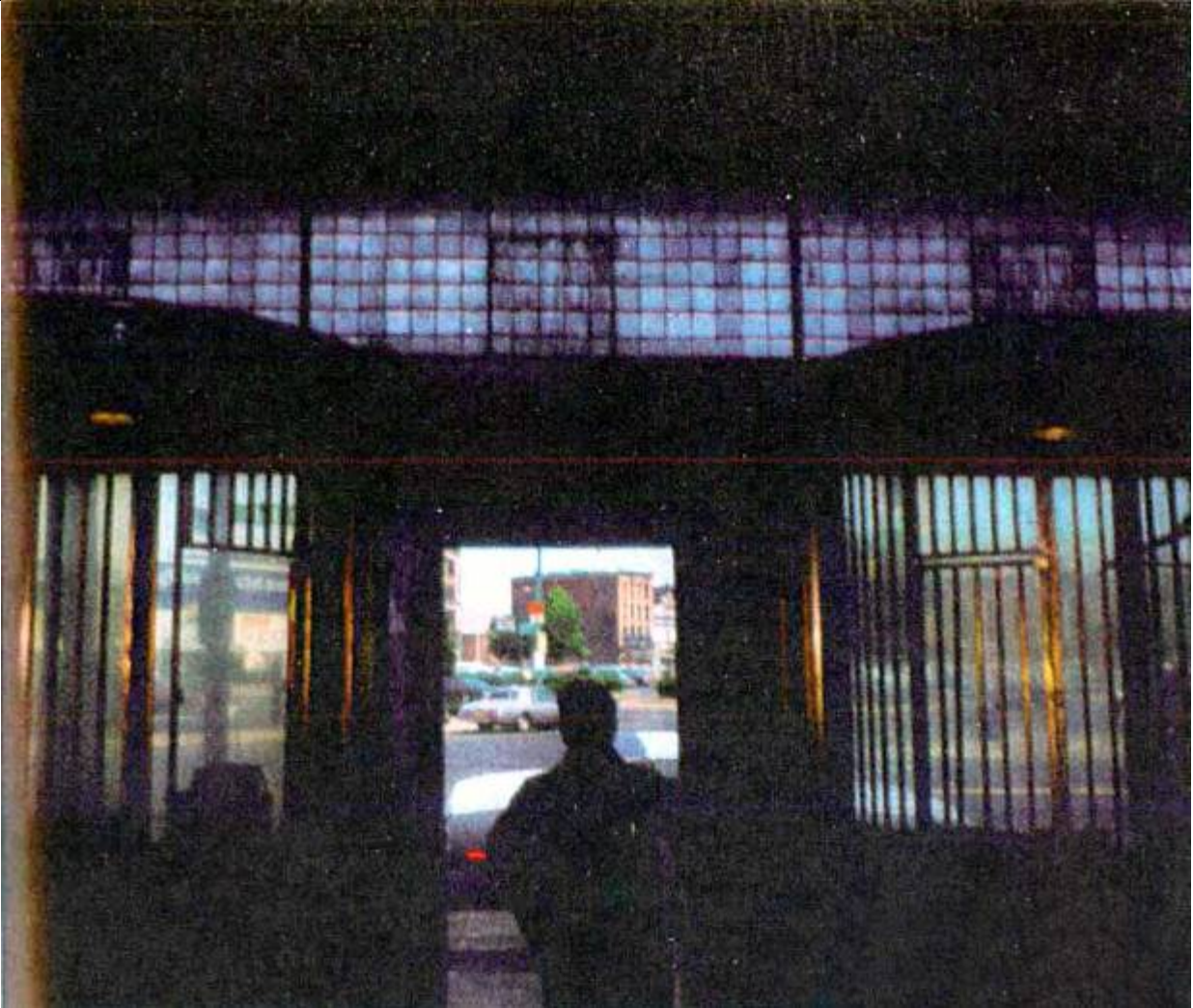
Interior of 87 Genesee retail space, looking north, 1980 (John Conlin, photographer) Notice how light-filled the commercial spaces were following the 1914 alterations done by Colson-Hudson. This image highlights the ample storefront display windows as well as the Luxfer prism transom above.
