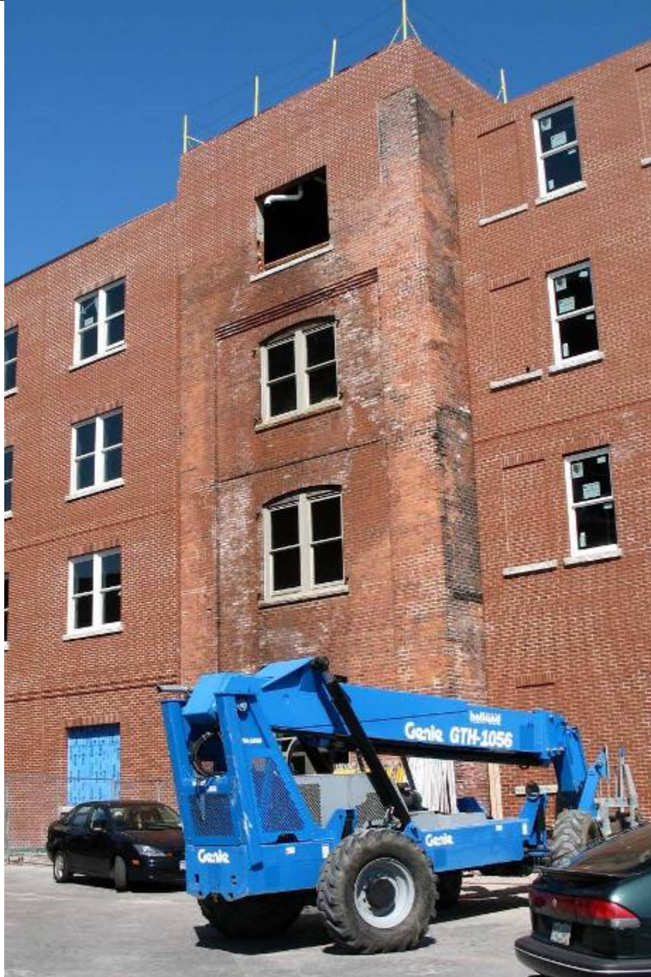
(11) 109-111 Genesee Street (south elevation)
