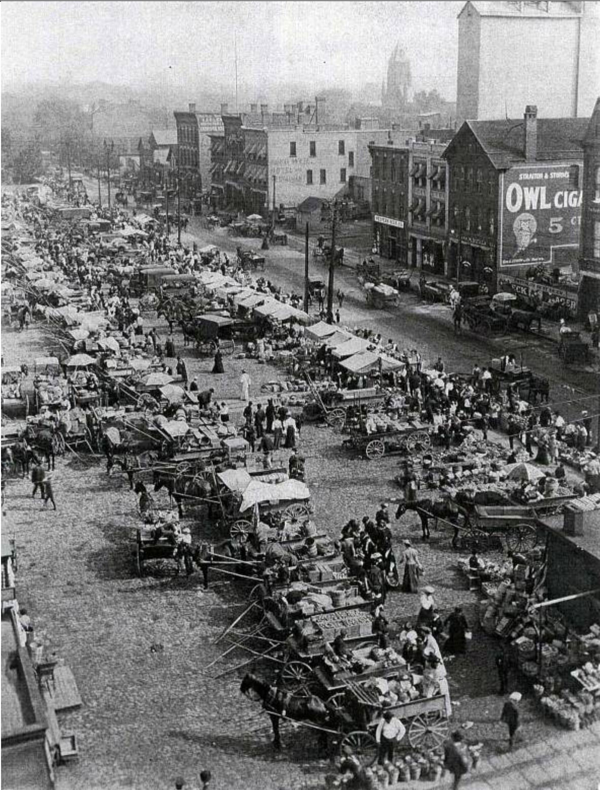
The Washington Market looking north-east along Ellicott Street, 1905 This view on a crowded market day shows the type of commercial neighborhood which had grown up around the Washington Market by the turn of the twentieth-century. The tall structure just visible in the upper right corner of the image is the Urban Roller Mills milling building.
