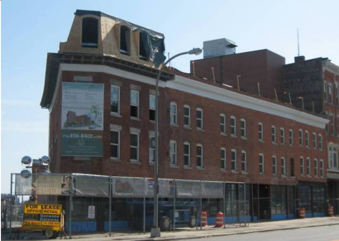
(9) 113-125 Genesee Street The H. Seeberg Building, ca. 1840s-1870s Contributing
