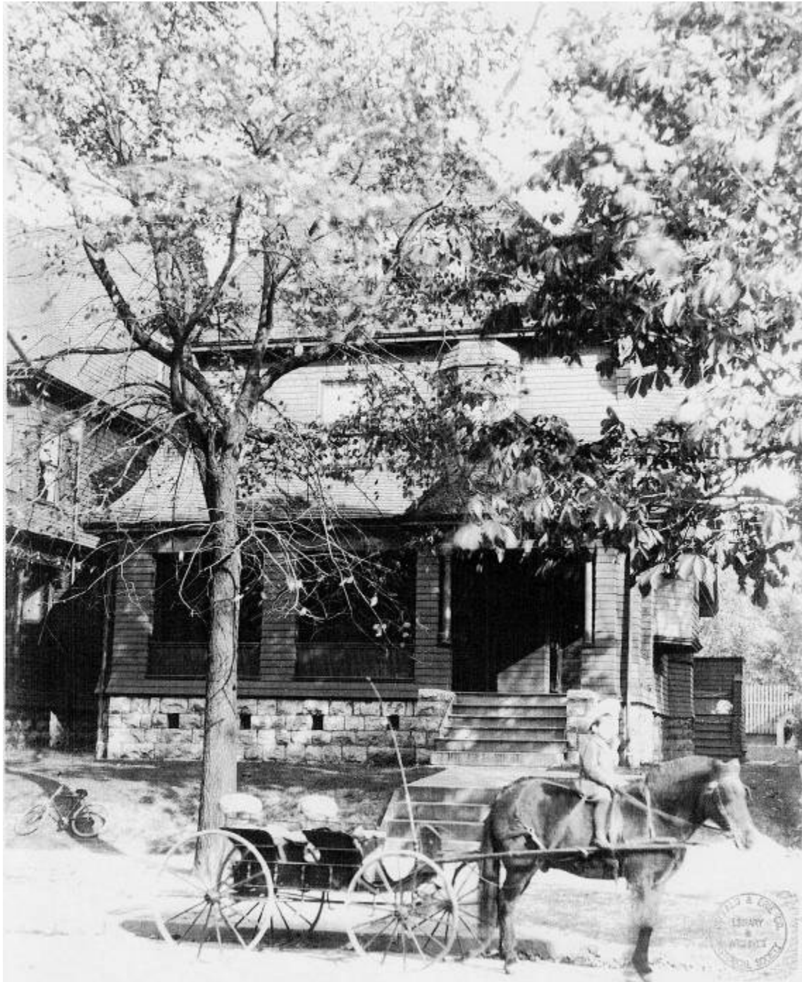
House at 27 Ashland Avenue (1904) Courtesy of BECHS
