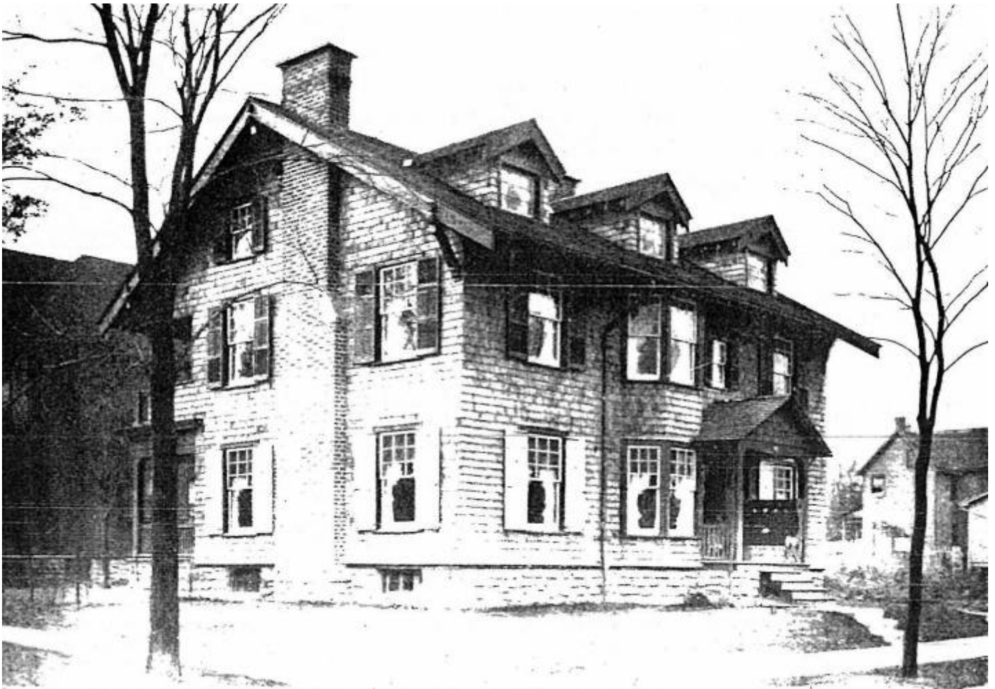
48 Dorchester Road, George F. Townsend, designer (1907) from The American Architect and Building News (April 27, 1907).
