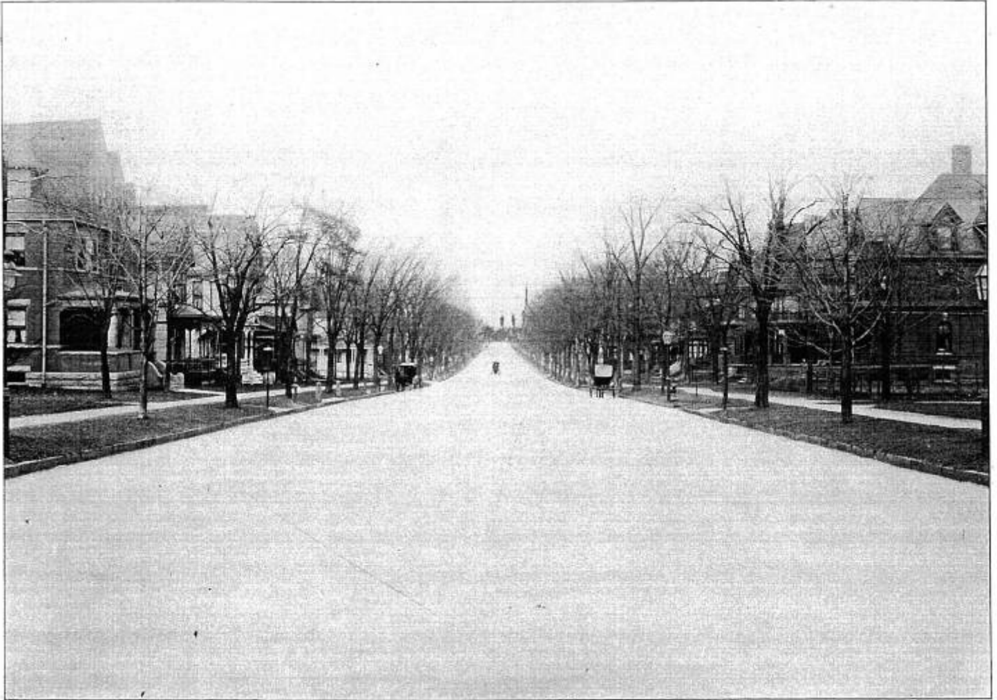
RICHMOND AVENUE, LAID WITH TRINIDAD ASPHALT PAVEMENT.
