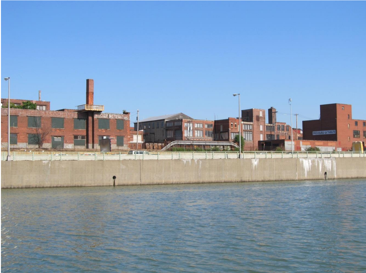
Looking southeast from the Black Rock Canal showing the Sterling Engine Company Buildings.
