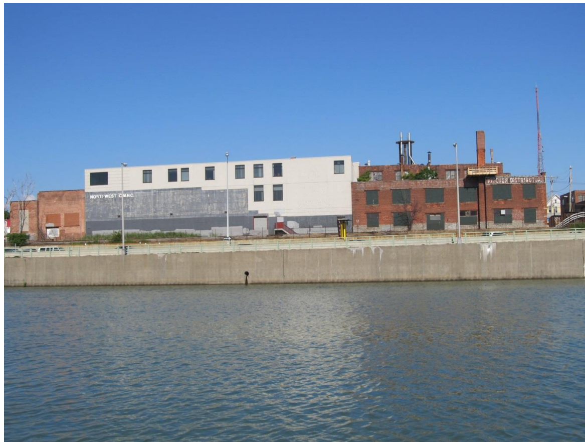
Looking east toward 1294 Niagara Street and 20 Auburn Avenue from the Black Rock Canal.
