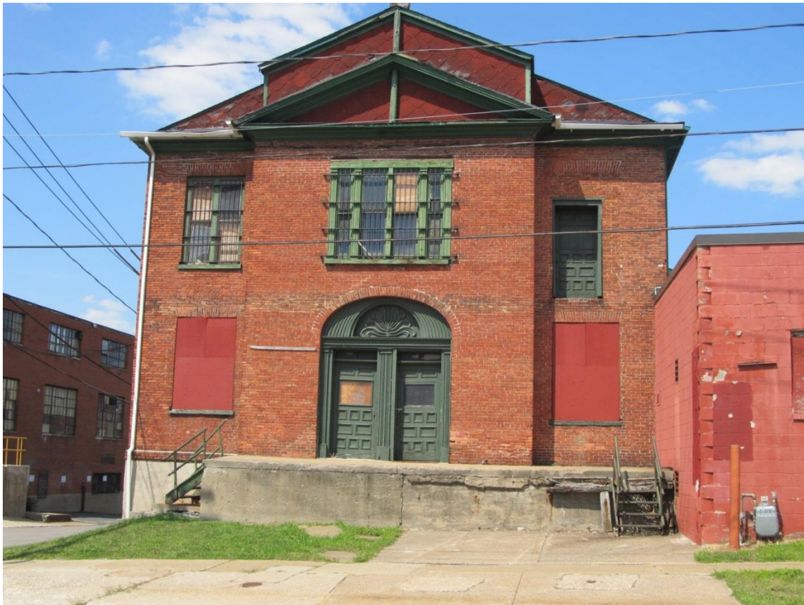
Looking north toward south elevation of The Union Meeting Hall – First Presbyterian Church of Buffalo.
