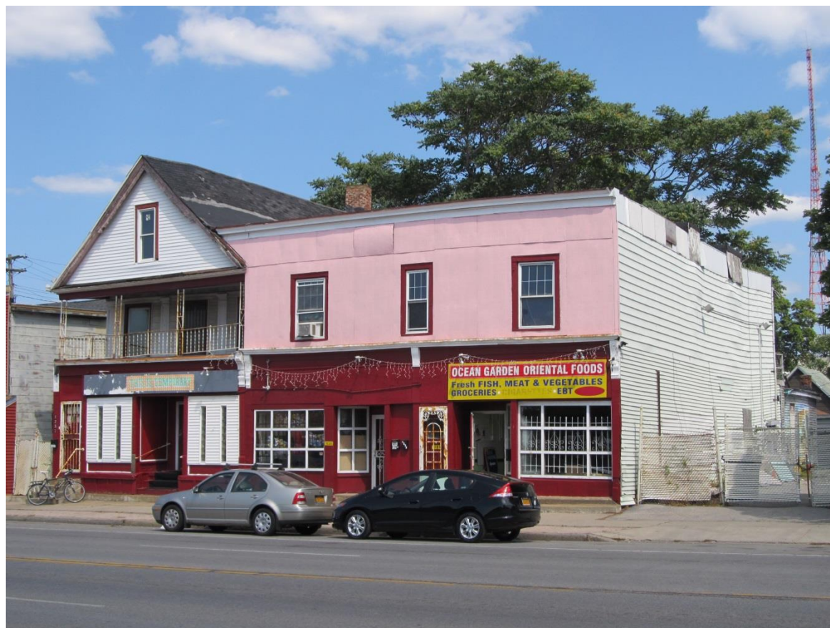
Looking northeast toward 1233 Niagara Street.
