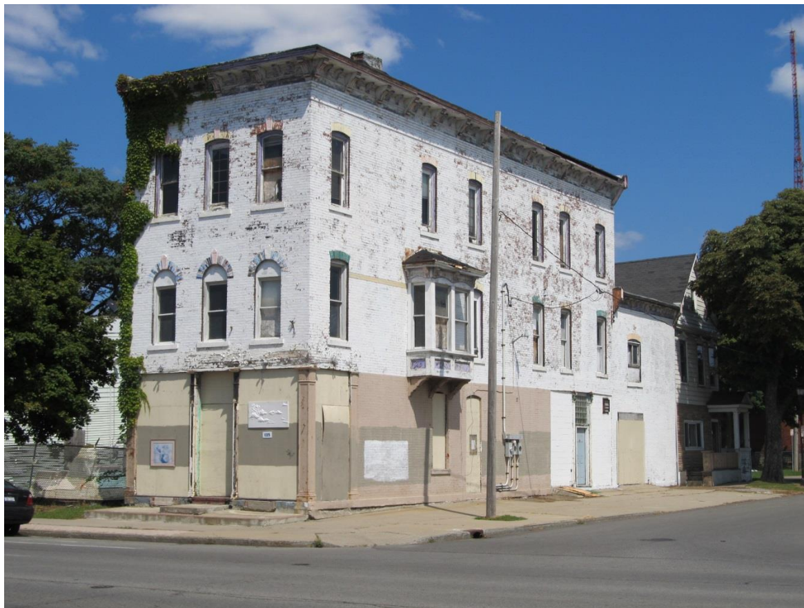
Looking northeast toward 1225 Niagara Street.
