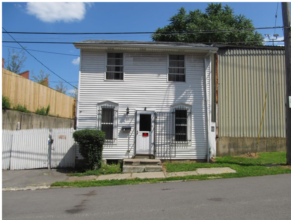
Looking east toward the residence at 19 Mason Street.
