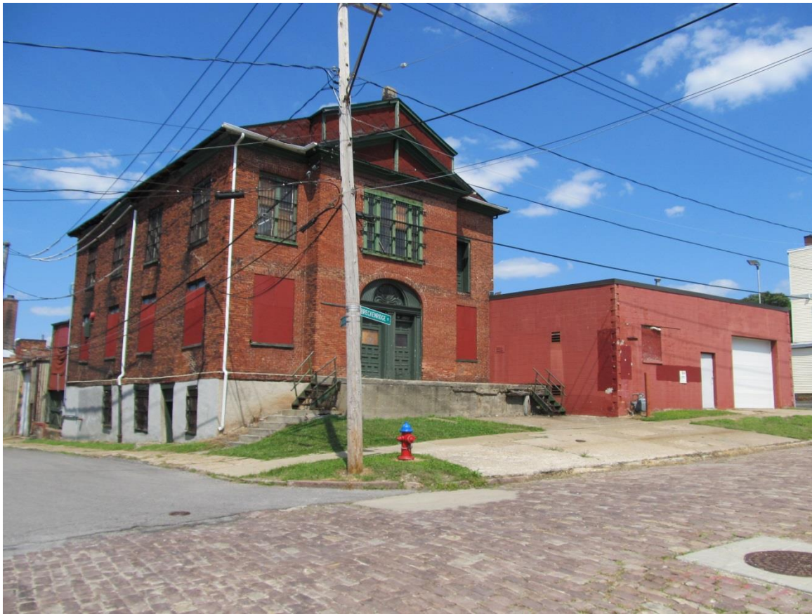
Looking northeast showing west elevation facing Mason Street and south elevation facing Breckenridge Street. The Union Meeting Hall – First Presbyterian Church of Buffalo. Note cobblestone street along Breckenridge Street.
