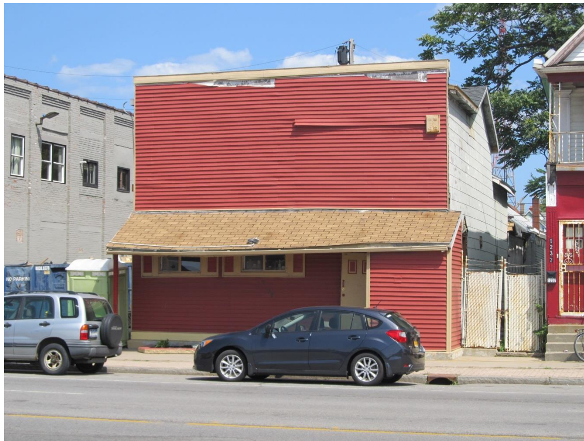
Looking northeast toward 1239 Niagara Street.
