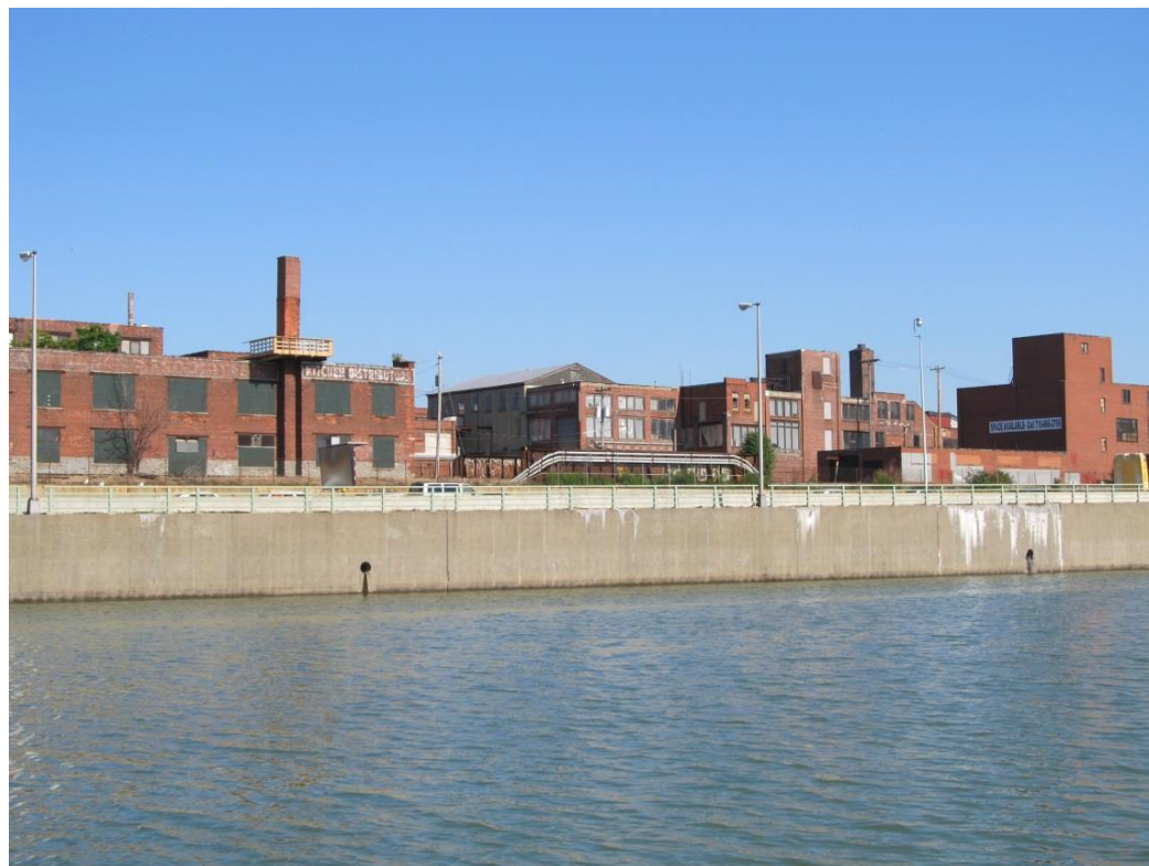
View of Black Rock Canal – Belt Line – Niagara Street Industrial Heritage District from Black Rock Canal.
