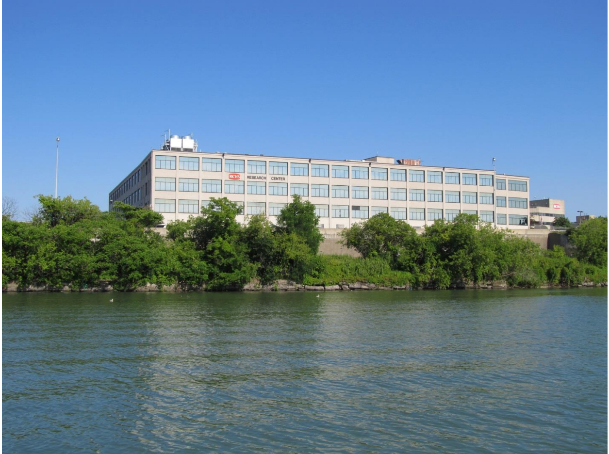
Looking southeast toward 1200 Niagara Street from the Black Rock Canal.
