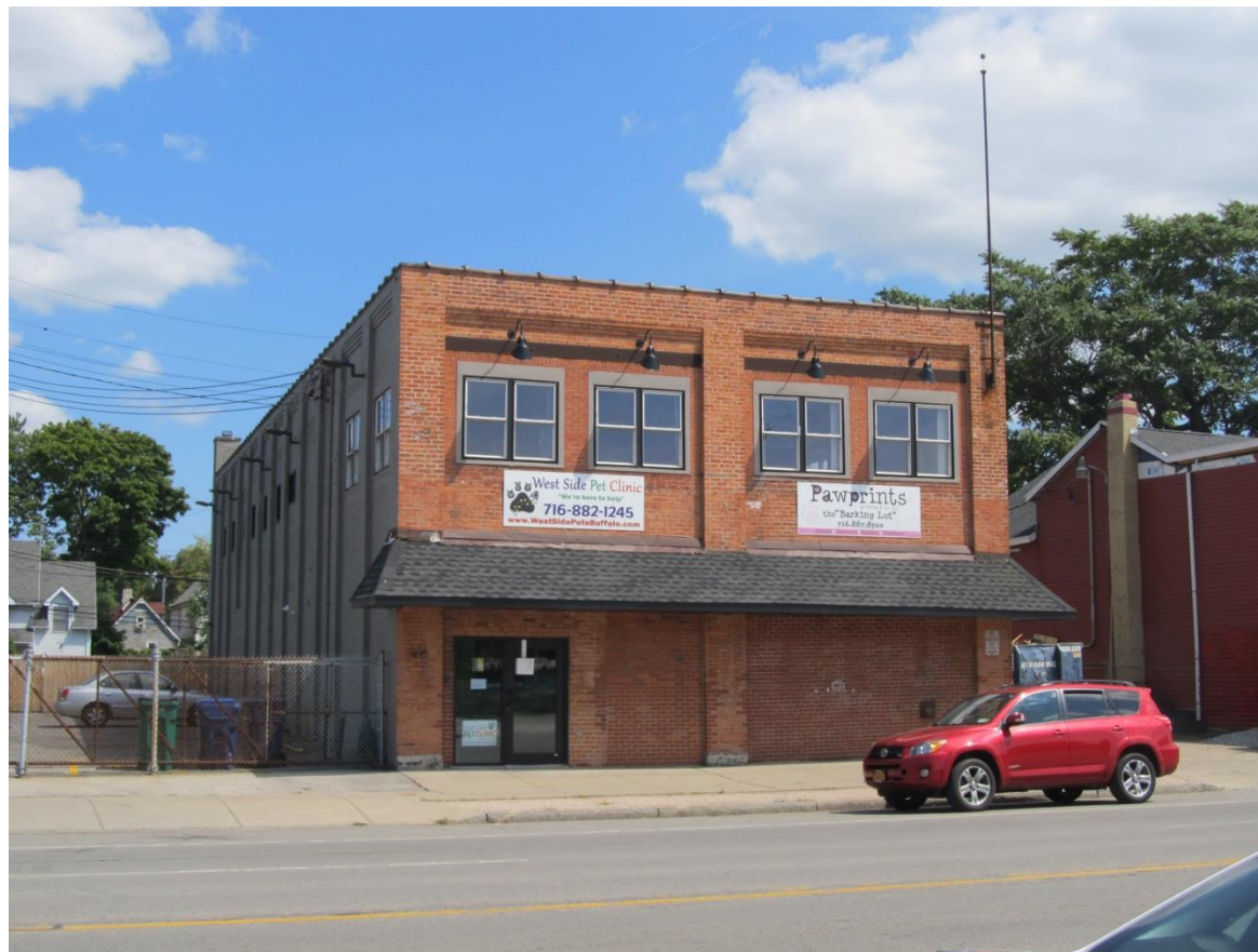
Looking southeast toward 1245 Niagara Street.
