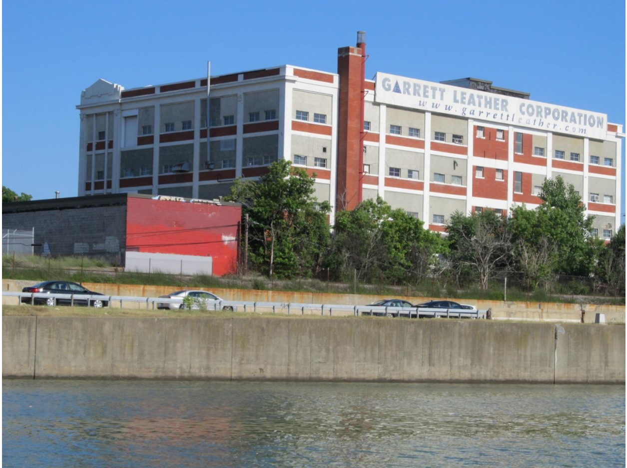
Looking southeast from the Black rock Canal toward 1360 Niagara Street.
