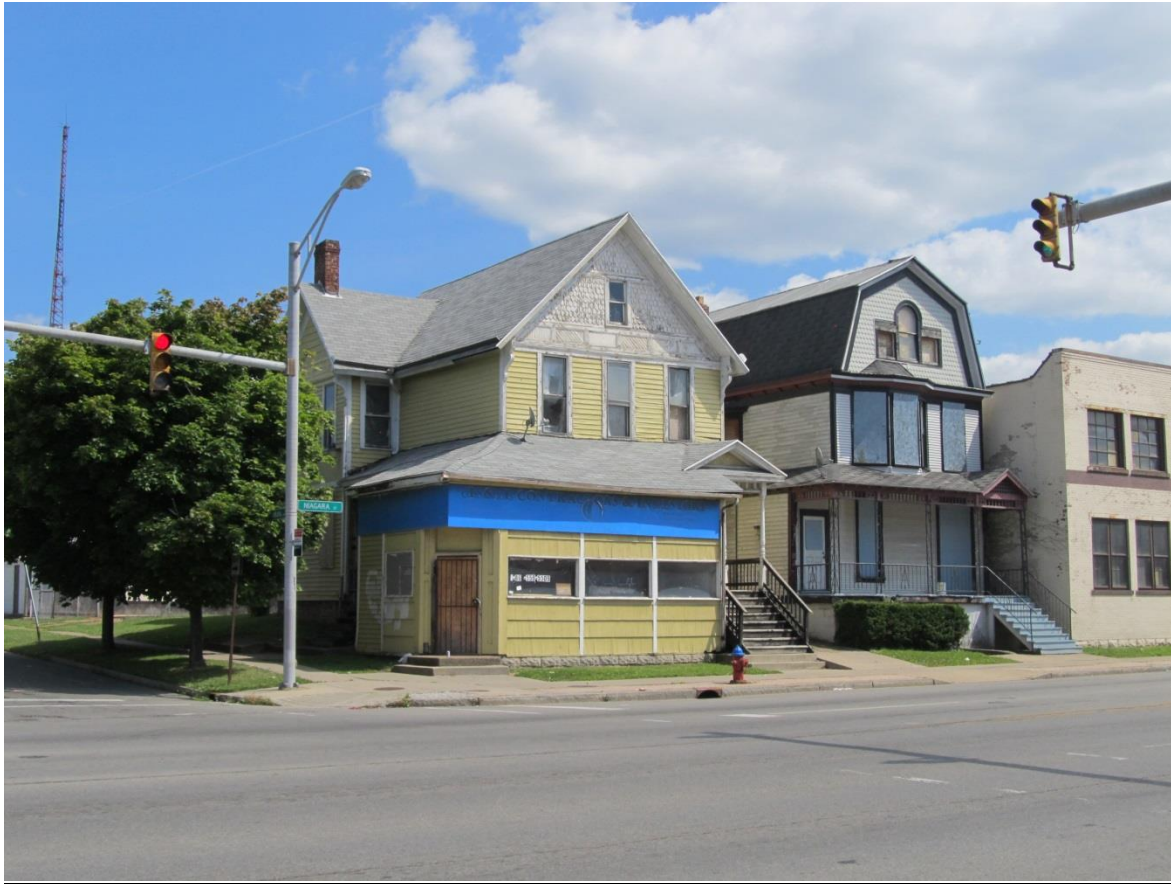
Looking southeast toward the residences at 1273 and 1277 Niagara Street.
