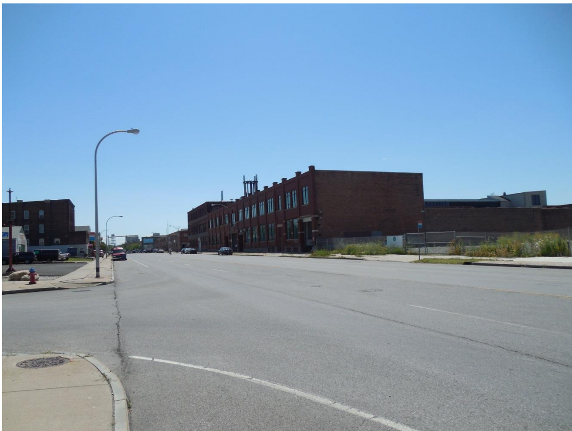
Looking southwest toward the Sowers Manufacturing Company, 1294 Niagara Street.
