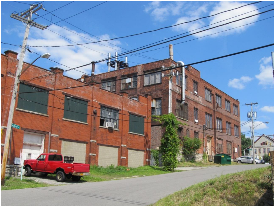
Looking northeast toward 20 Auburn Avenue and 1280 Niagara Street from Auburn Avenue – Buffalo Gasoline Motor Company.
