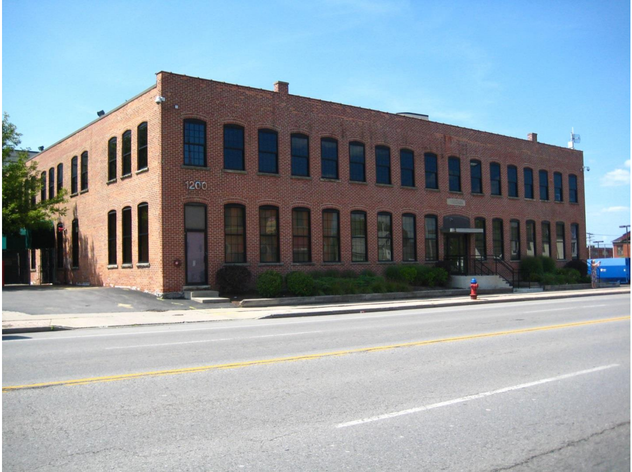
Looking northwest from Niagara Street toward 1200 Niagara Street.
