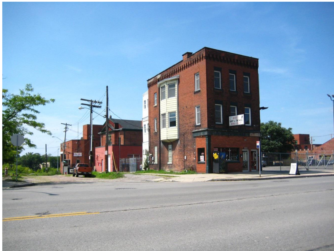
Looking northwest toward 1226 Niagara Street. Breckenridge Street, with the Union Meeting Hall – First Presbyterian Church and Sterling Engine Company are visible to the west.
