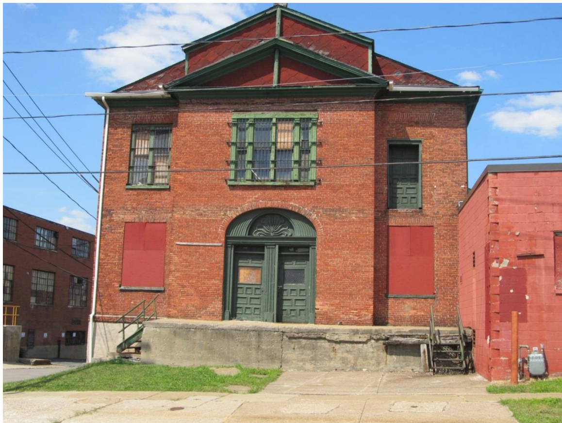
Looking north toward south elevation of The Union Meeting Hall – First Presbyterian Church of Buffalo.
