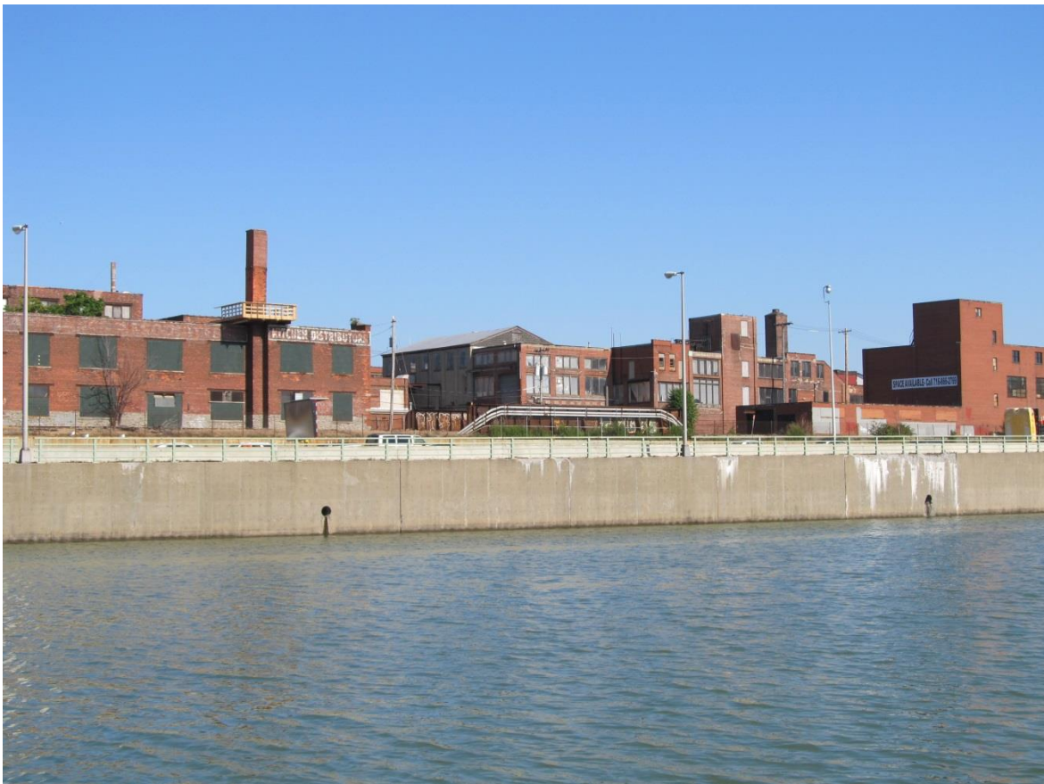
Looking southeast from the Black Rock Canal showing the Sterling Engine Company Buildings.
