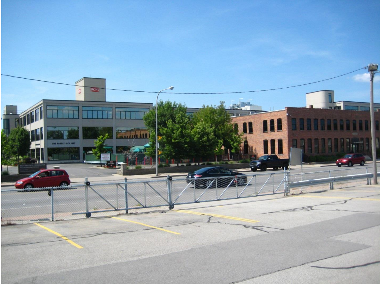
Looking northwest into 1200 Niagara Street from across Niagara Street.
