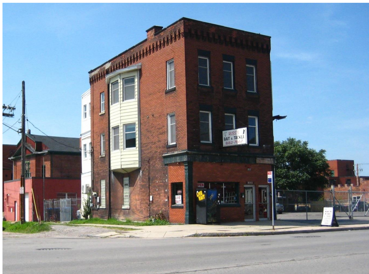
Looking northwest toward 1226 Niagara Street.
