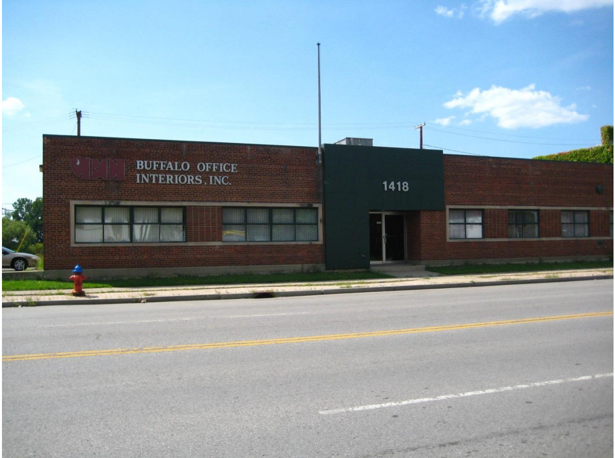
Looking northwest from Niagara Street toward 1418 Niagara Street.
