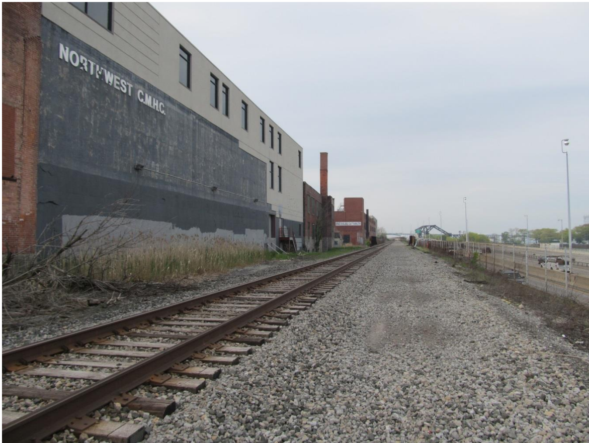
Looking southeast toward 1294 Niagara Street from Belt Line.
