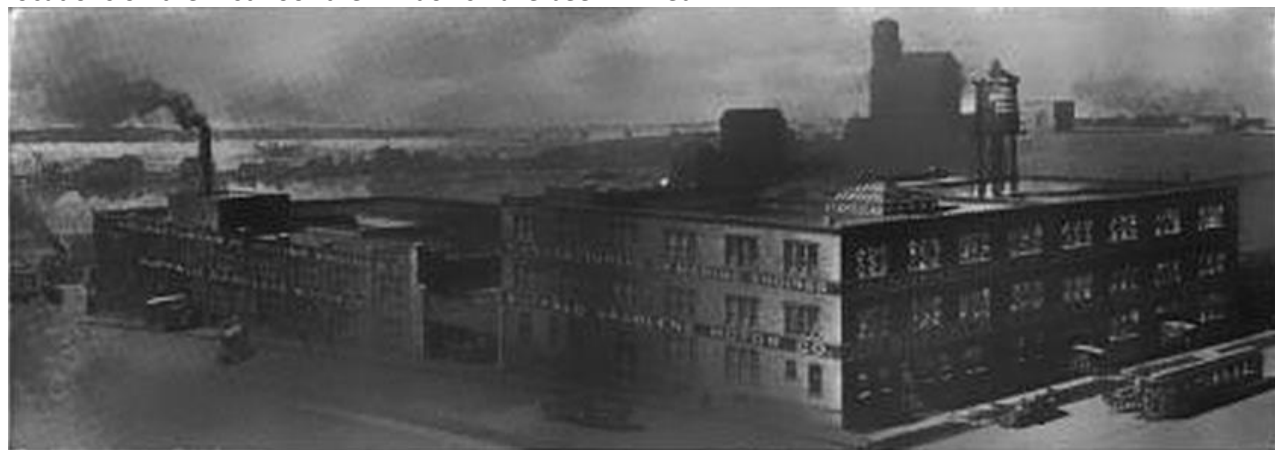
The large and well equipped factory where the Buffalo marine engines are built.
