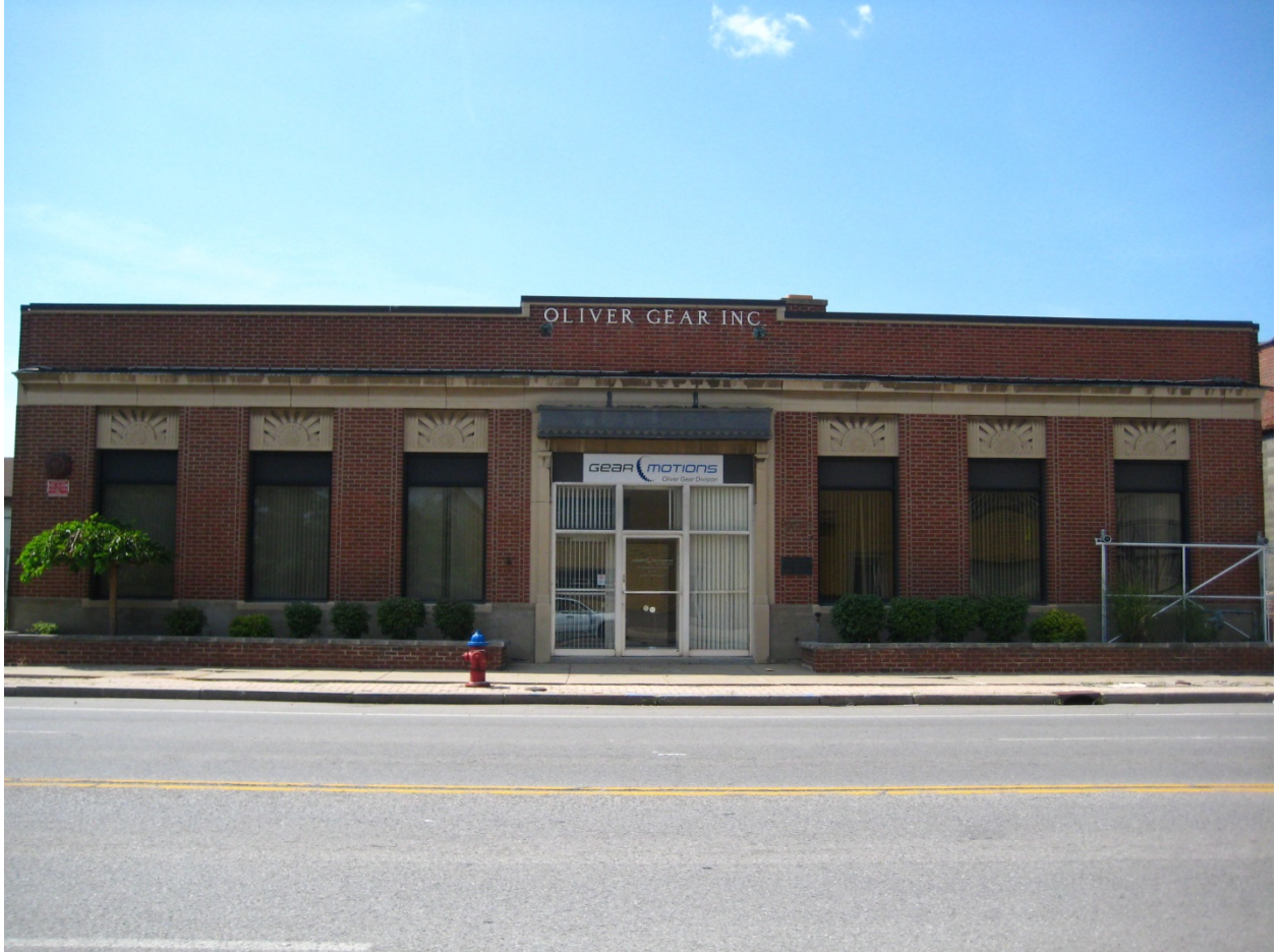
Looking west from Niagara Street toward 1114 Niagara Street.
