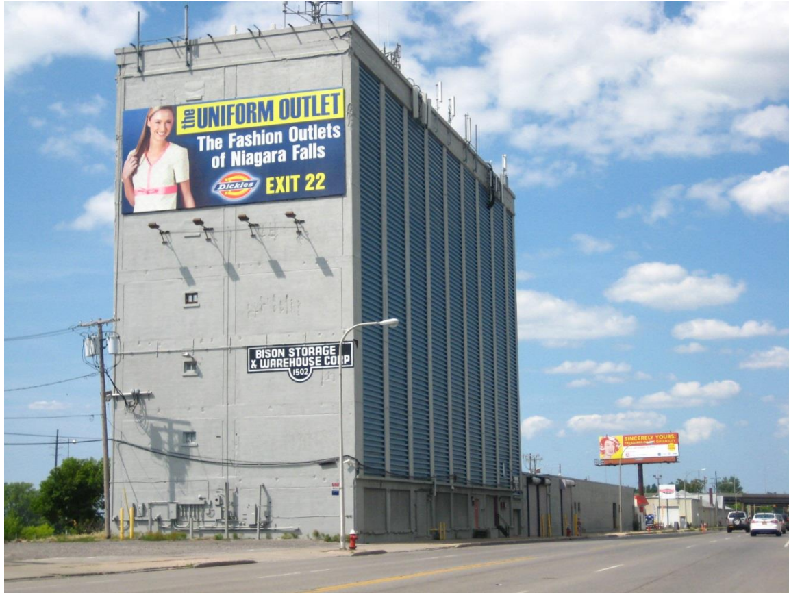
Looking northwest from Niagara Street toward 1502 Niagara Street.
