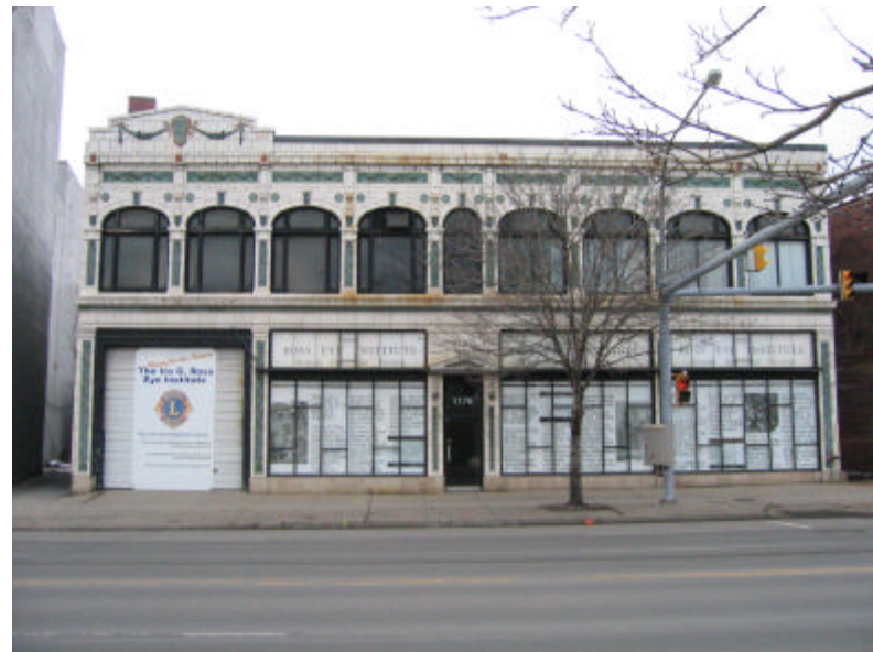
The Ross Eye Institute on Main Street, across from the intersection with Dodge Street, is a colorful example of the mixed-use buildings common to Midtown.
