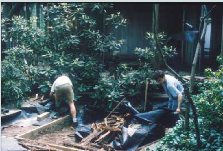
Pool under repair, late 1990s. Courtesy JRC.
