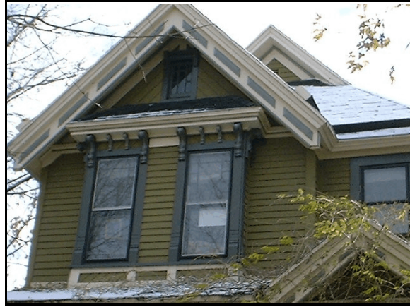
3F - 248 Lexington Ave. Detail - same paneled verge board as 14 th Street and 164 Fargo.
