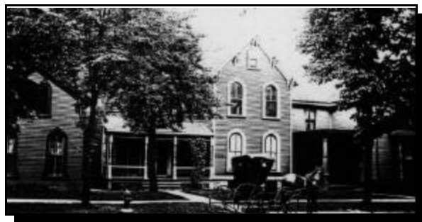
497 Porter (left), home of Richard Caudell, built circa 1864. (Demolished, date unknown.) Note horse and buggy.
