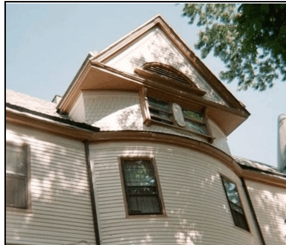
3N - 314 Hudson Street, gable detail on western elevation (Plymouth Ave.).
