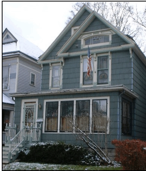
3H - 44 Orton Place. Similar gable window to 478 Connecticut Street and ancones as found on 11 Plymouth Ave. Circa 1887.
