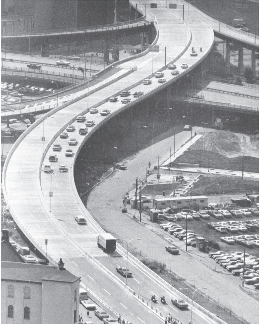
Figure 6: The renovated Skyway opens, 1976. Buffalo Courier Express Library Collection, Courtesy, E. H. Butler Library Archives, Buffalo State College.
