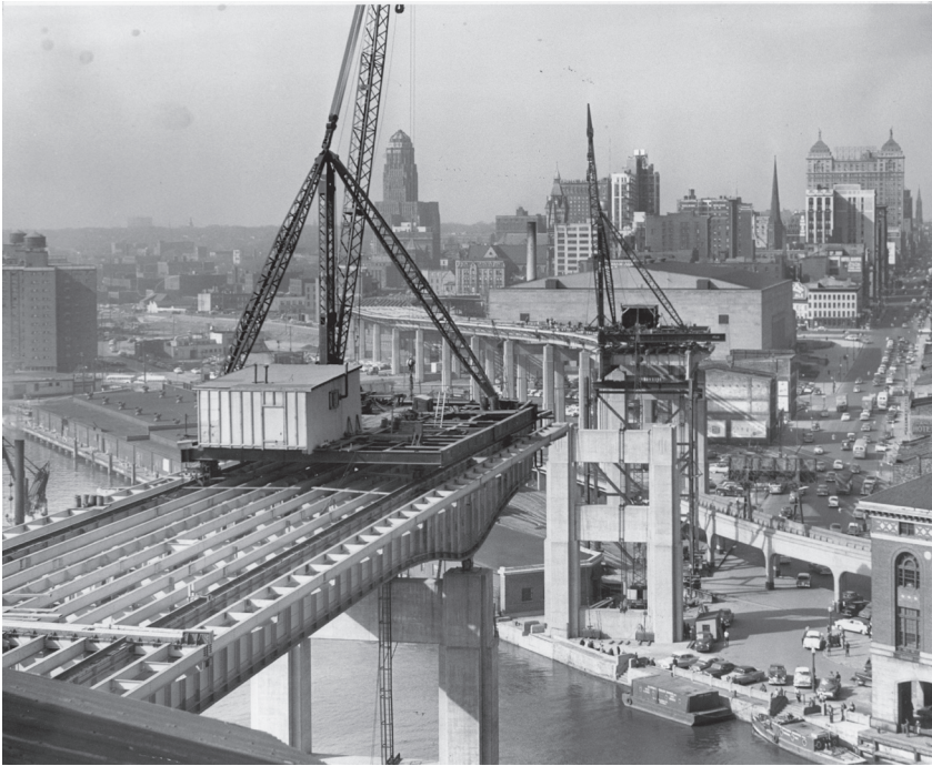
Figure 5: The Skyway under construction, April 14, 1955. Courtesy, Buffalo and Erie County Historical Society.
